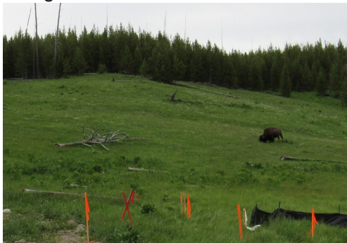
Local wildlife keeps an eye on this construction project in Yellowstone National Park.
